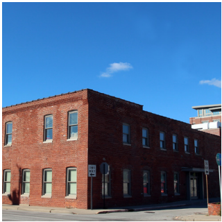
The Sol Center
